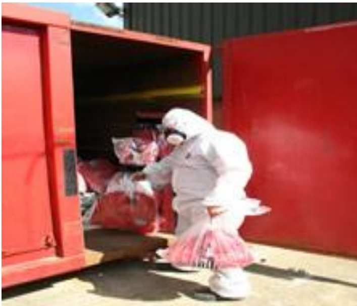
Double bagged waste being placed in lockable skip on site
